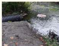
South Main St. near railroad bridge
