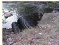
South Main St. near railroad bridge
