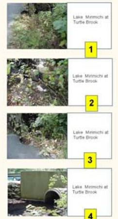
Lake Mirimichi at Turtle Brook: ① concrete pipe in stone and cement headwall. Some exposed rebar and part of the lower headwall has collapsed into Turtle Brook. The road surface has sloughed and eroded near this structure. The gravel base is compromised in spots and runoff can drop directly into the waterbody from the road at this point. Turtle Brook had a steady flow but silt of silt.
