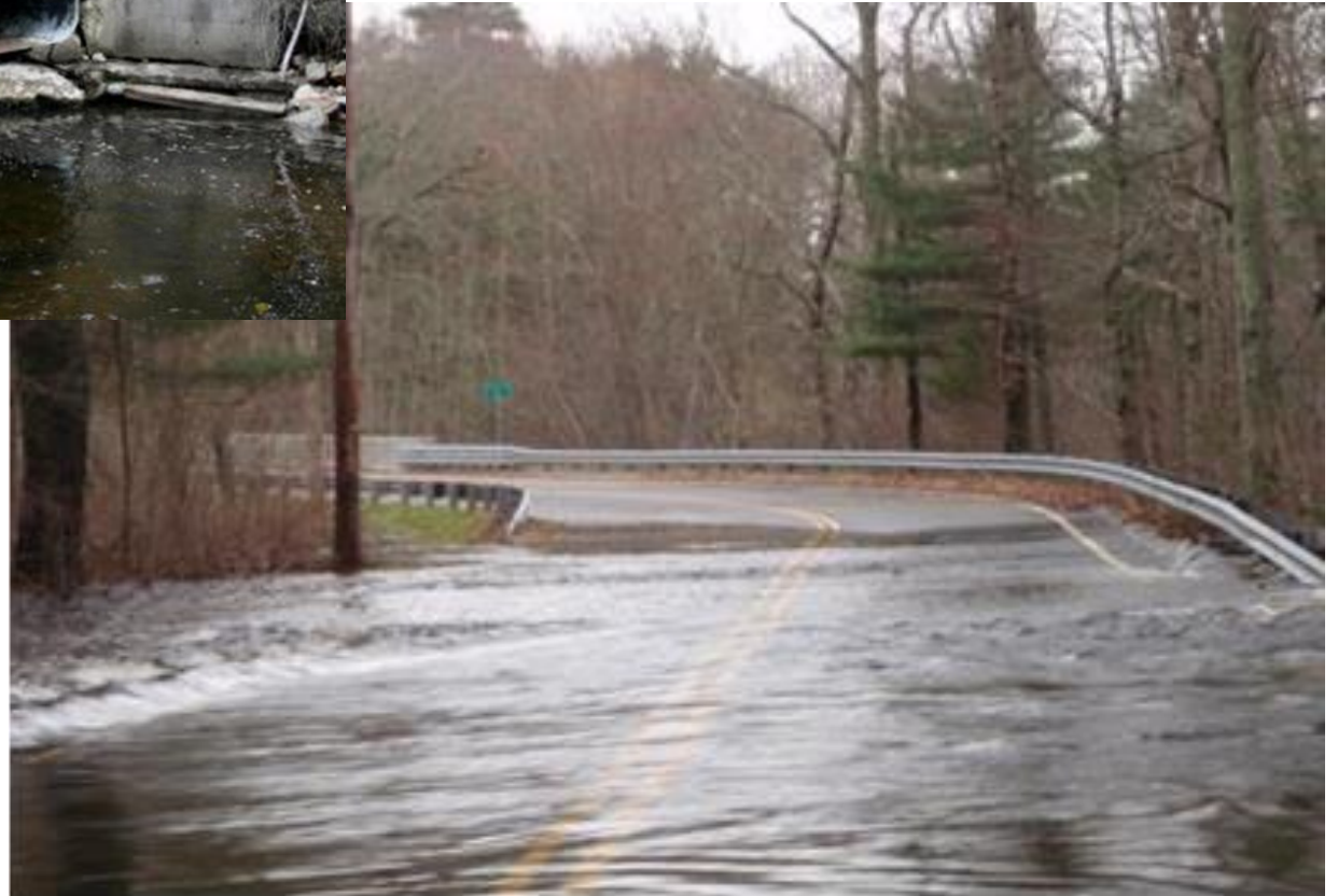
CRANE STREET, NORTON MA, 2010 FLOODING
