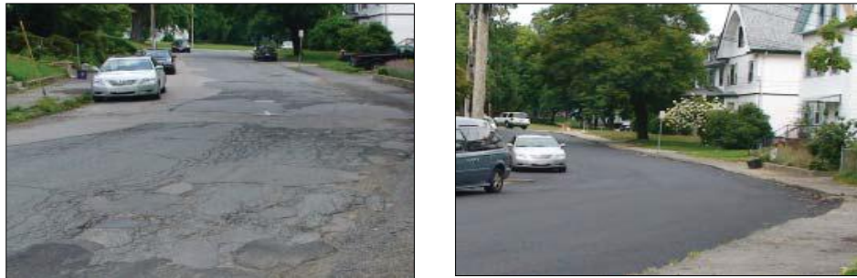
Figure F-1: Pavement conditions before and after repairs
