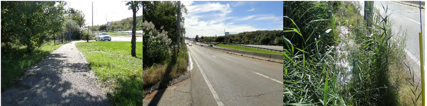
Figure 4: North Attleborough Marketplace Sidewalk End Conditions
