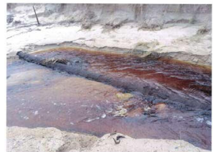
Exposure of Water Main at Pease's Point and Point Connett during June 2013 storm
