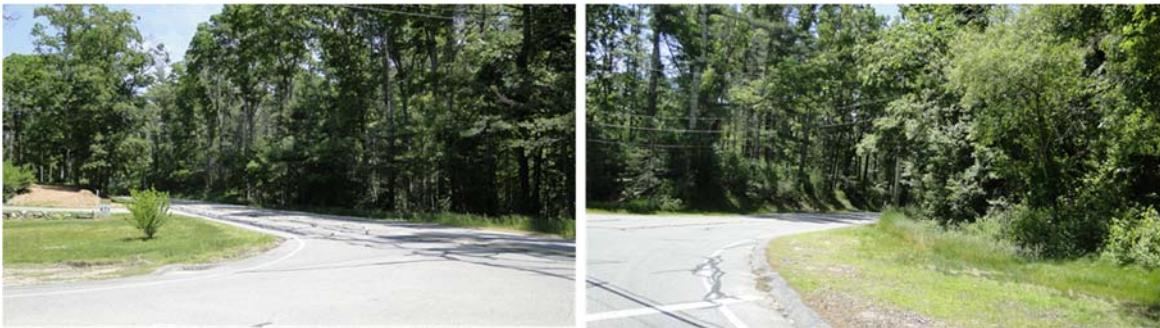
**Figure 4: Sight Distance at the Stop Sign at the Southbound Approach**
