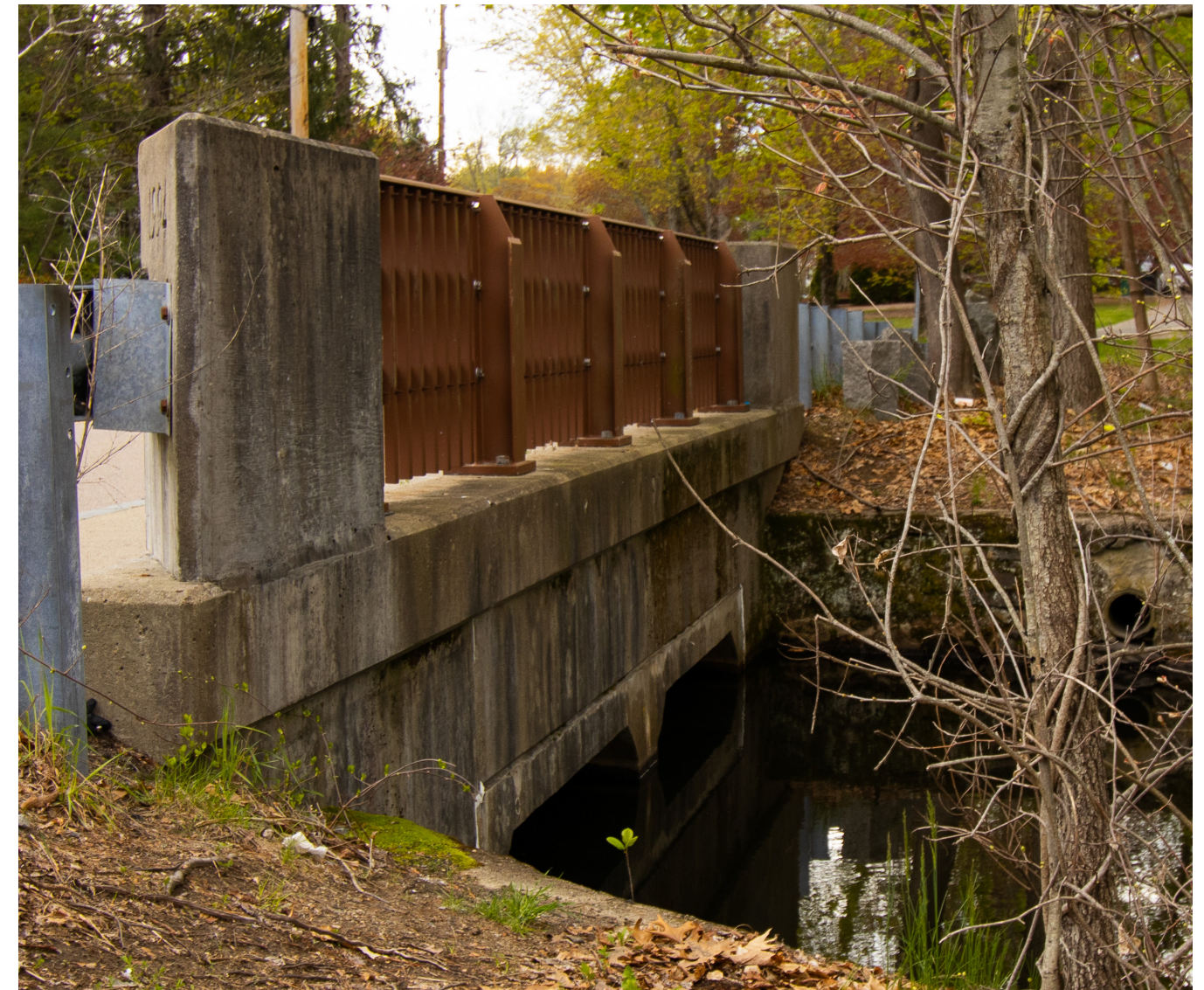
Image 12: A culvert along the Ten Mile River [Taylor Perez/SRPEDD]
