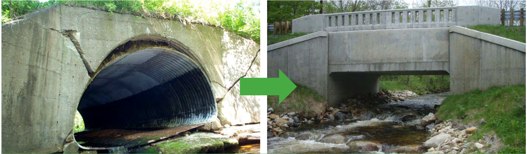
McInerney Road over Shaker Mill Brook in Egremont, MA
