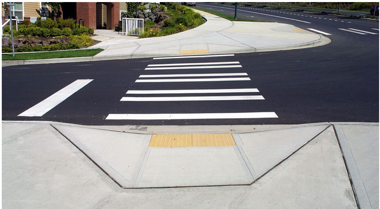
Figure 4-4: Sidewalk with a wheelchair ramp and tactile warning panel
