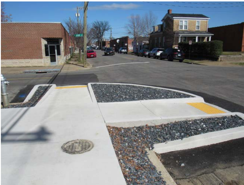
Figure 4-13: Curb ramps with tight corner radius in Richmond, Virginia
