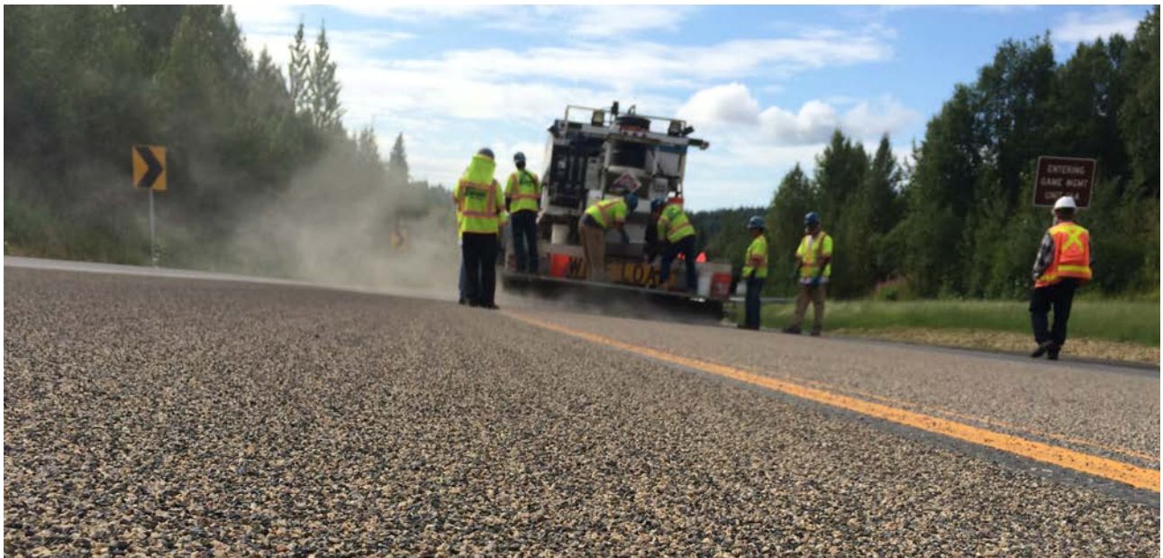
Figure 4-31: Workers installing high friction surface treatment on a road
