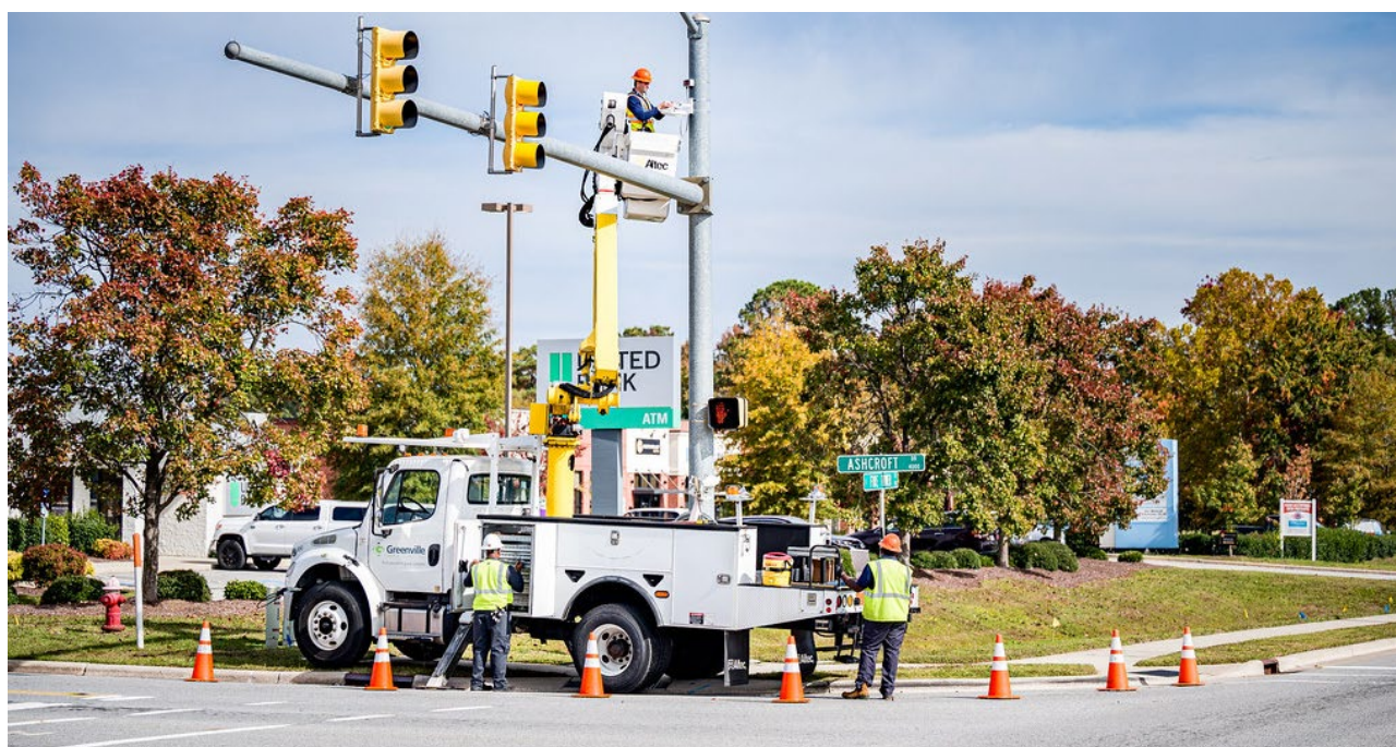
Figure 4-12: Workers updating signal equipment
