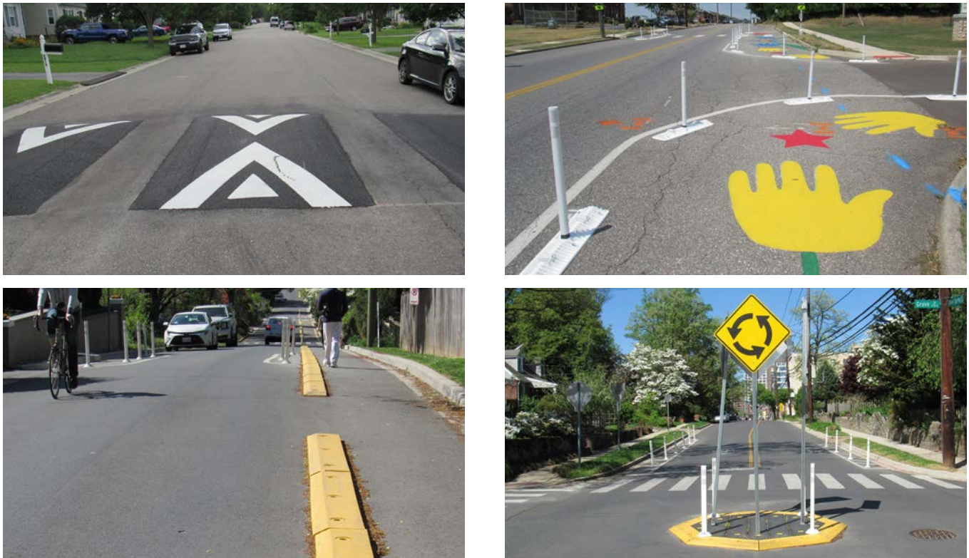
Figure 4-32: Examples of Pop-up Traffic Calming - Speed Humps (upper right), Corner Radius Re-education (upper left), Temporary Curb (lower left), Temporary Roundabout (lower right)
