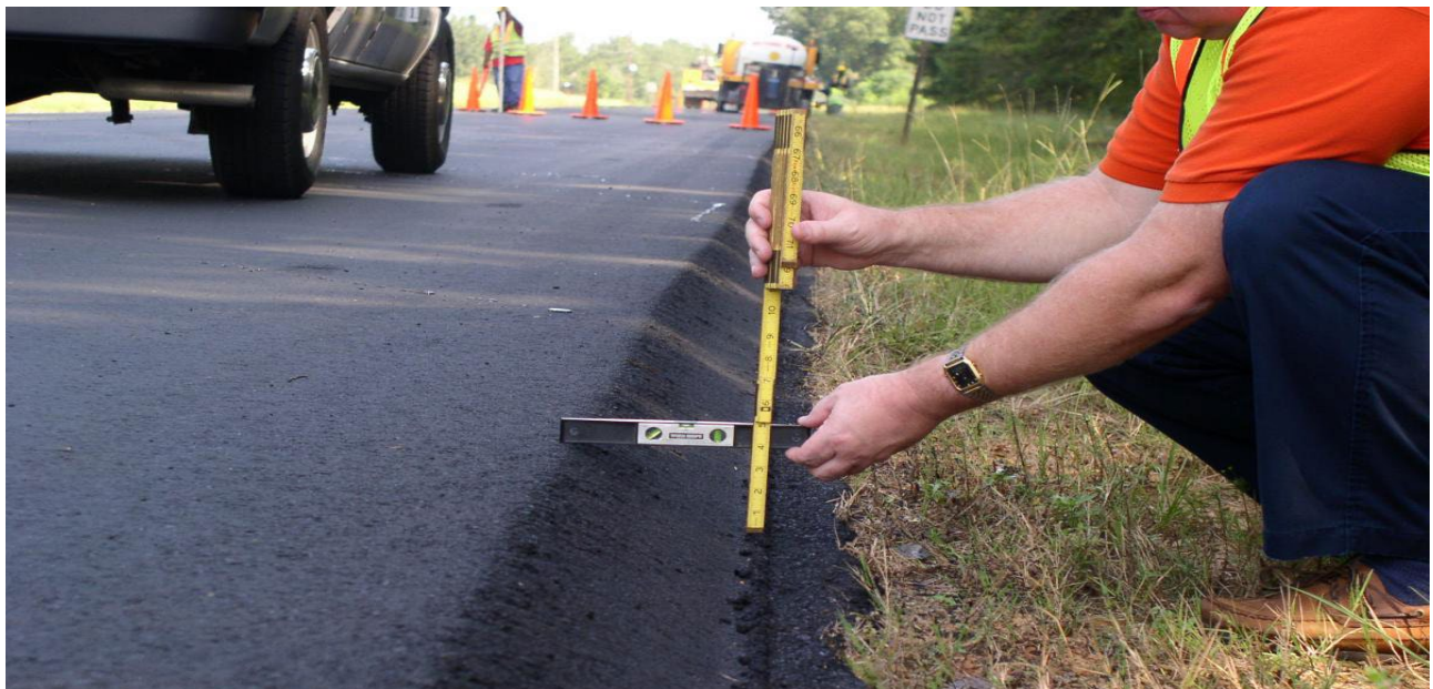
Figure 4-30: A Worker measures the edge of the pavement
