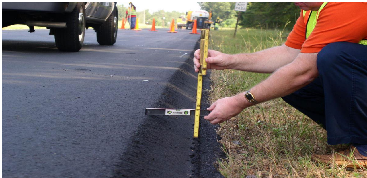
Figure 4-21: A Worker measures the edge of the pavement
