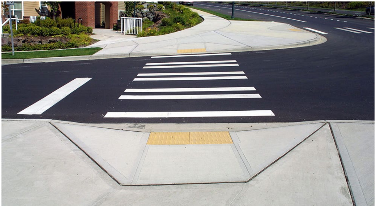
Figure 4-3: Sidewalk with a wheelchair ramp and tactile warning panel
