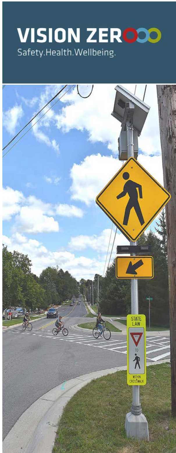
Figure 1-1: Picture showing cyclists using a crosswalk with high visibility markings and a rectangular rapid flashing beacon.
