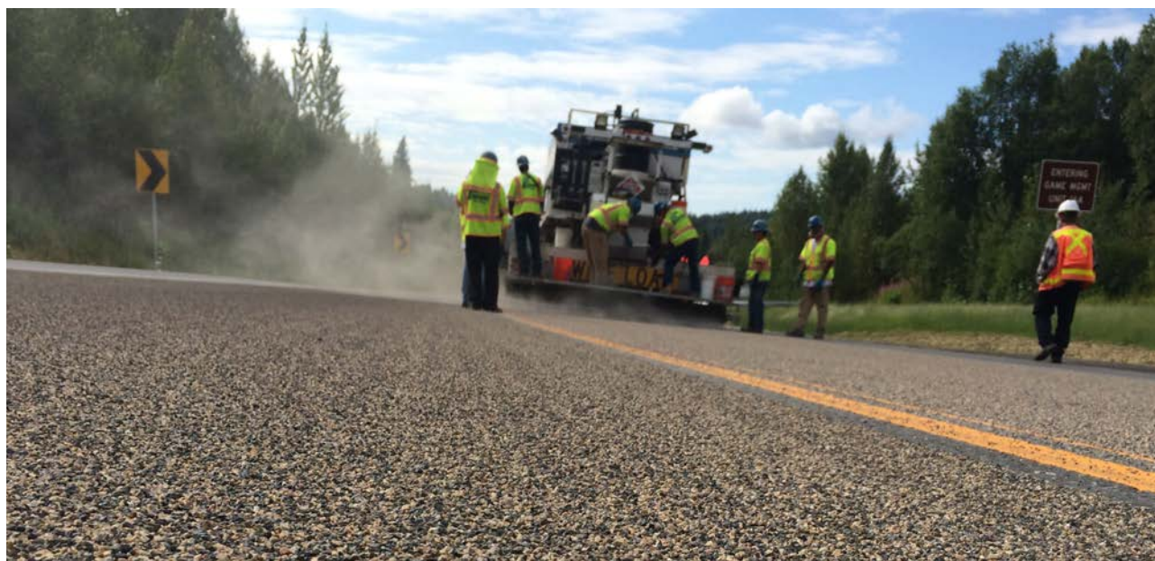
Figure 4-22: Workers installing high friction surface treatment on a road
