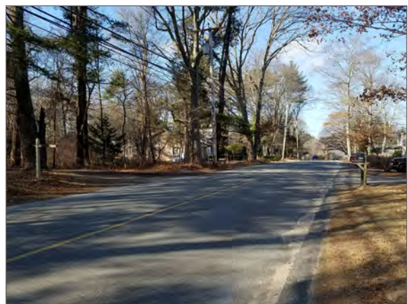
Figure 3: Thickly settled area on Reservoir Street without bicycle and pedestrian facilities.
