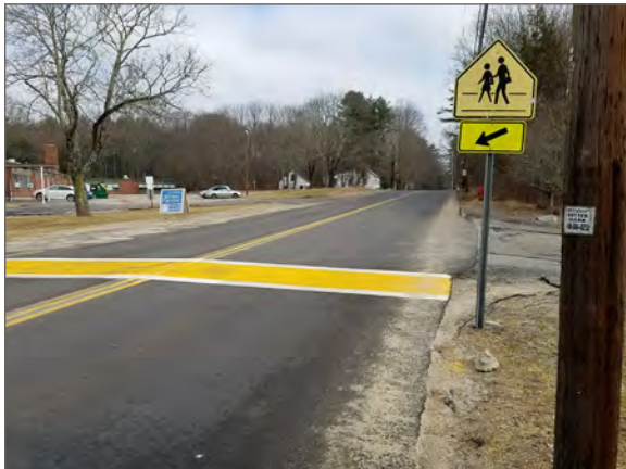
Figure 9: “Solid” type crosswalk on Plain Street at the L.G. Nourse Elementary School.
