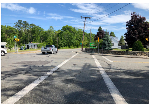
Figure 15: “Standard” style crosswalk on Wood Street
