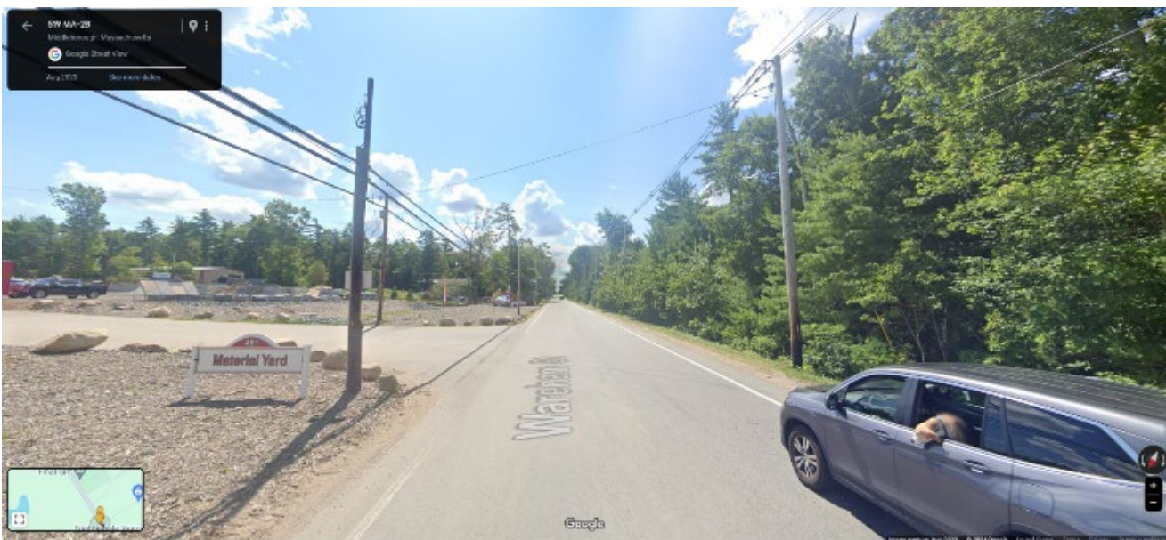
Figure 13: Utilities on both sides of the road in Middleborough
